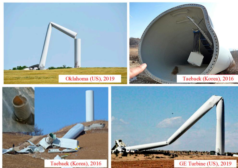
**Figure 1.** Failure of wind towers.
